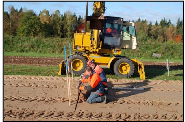
Fibre board being buried
