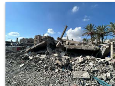
Start of the UNMAS- UNDP Debris Management Pilot Project, Sept 2024
